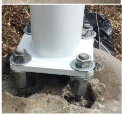
1-8 UNC Galvanized Female Thread 1.375" of internal thread.
