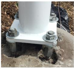
1-8 UNC Galvanized Female Thread 1.375" of internal thread.
